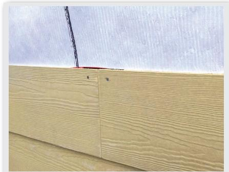
**STEP 1:** Install the first pieces of lap siding without nailing the end near the butt joint.
